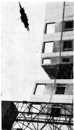
Fig. 5. Transportation of prefabricated piping.
